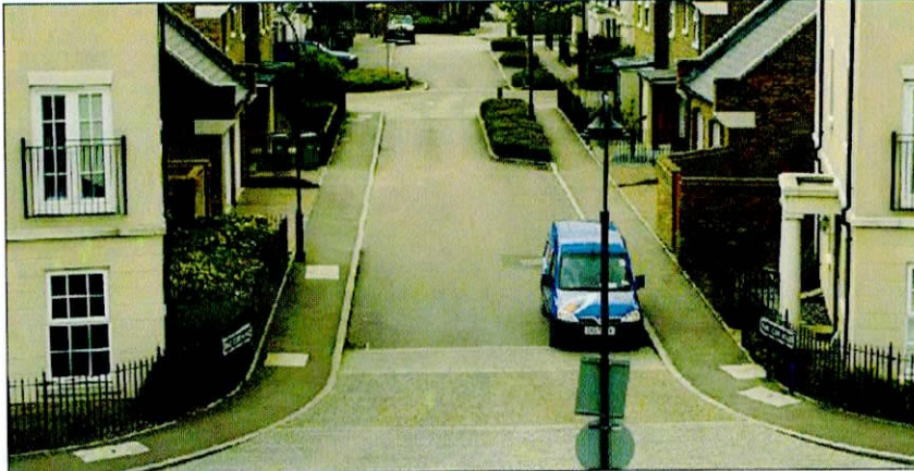
Figure 4.71: An example from Ingress Park, Kent, UK, of how the path and speed of a vehicle is altered within a low speed environment through the use of vertical and horizontal deflections (and material changes).
