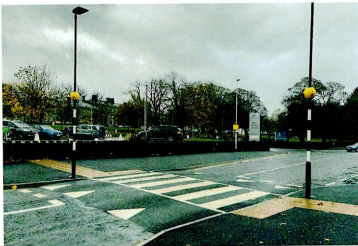
Image 5.3: Raised zebra crossing with Belisha Beacons
